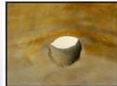
Full drain outlets drilled out removing the liner
